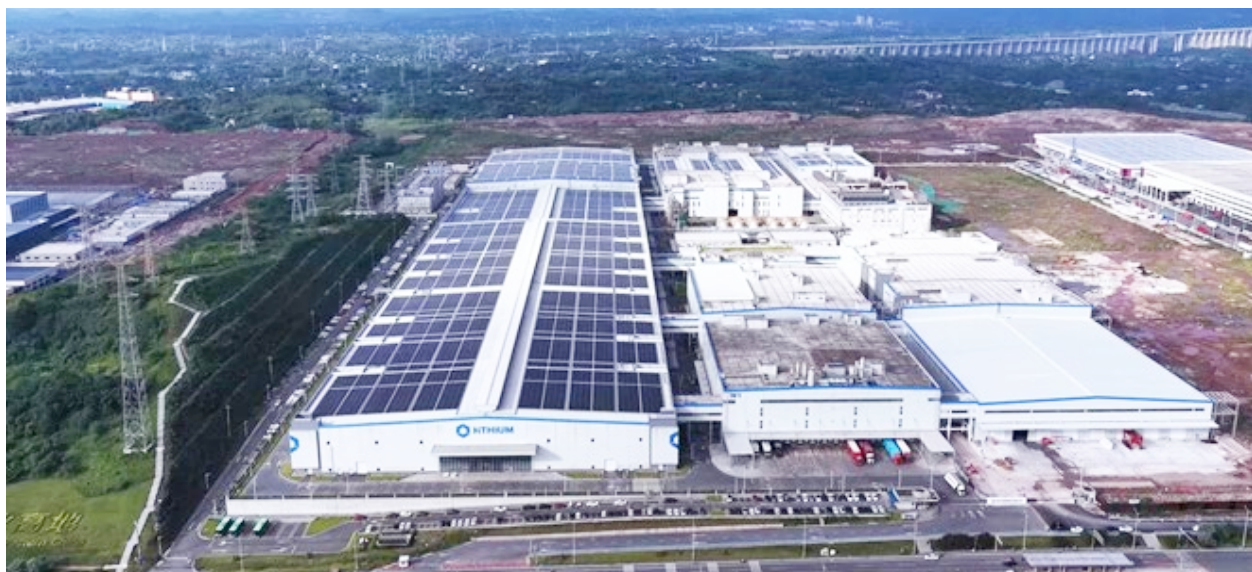
Hithium Chongqing Base
